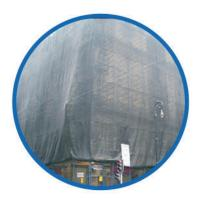
**FABRIC FOR BUILDING FACADE:** The Mesh for Facades are used to provide a better appearance and privacy to your projects, also achieving a cooler, ventilated and safe work environment.
